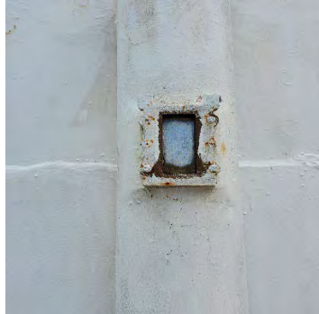
Foggy Tank Level Gauge
